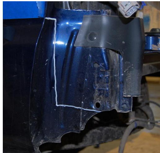
Figure 2. Rear bumper relief cut. Drawn 1 inch higher than first cut should be.
