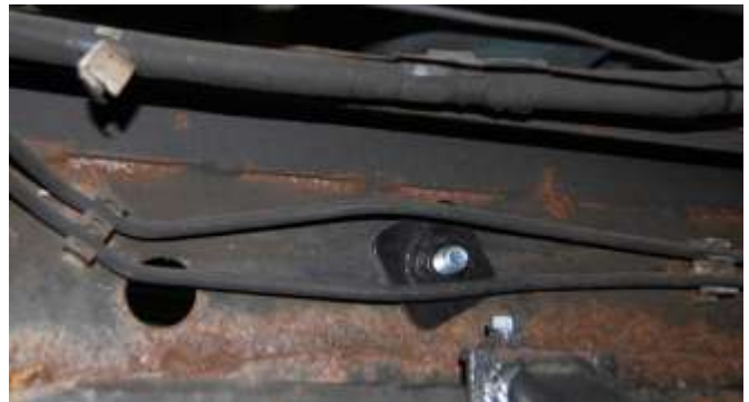
Figure 3. Inside driver's side frame rail, behind transmission cross member, brake line modification.
